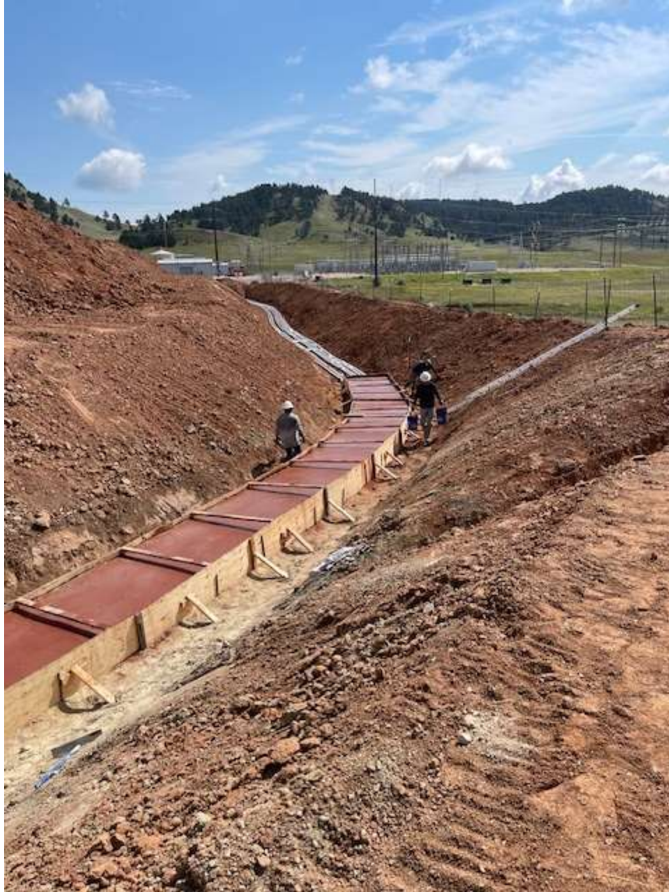
Poured duct bank 8/25/2025
