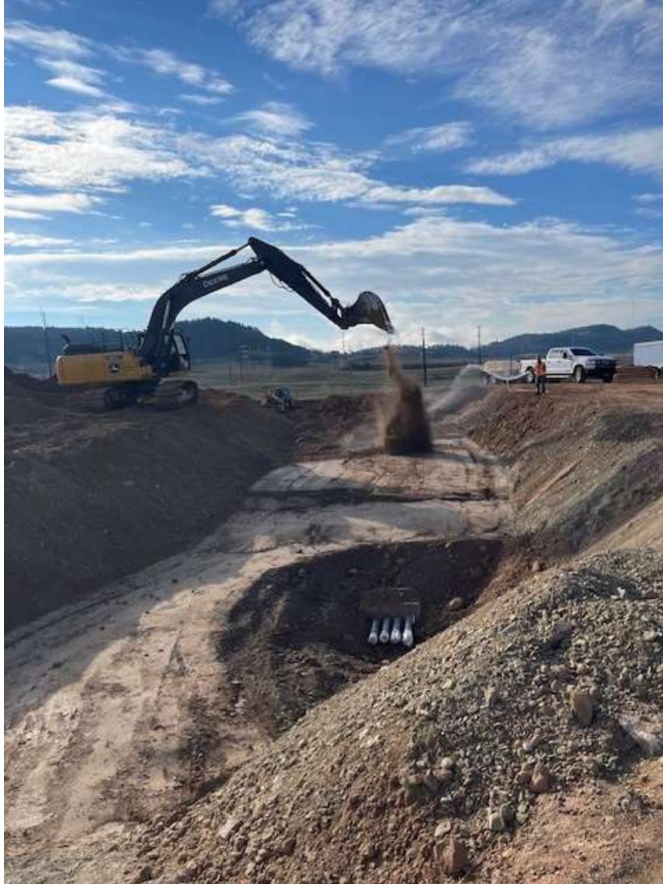
Trench backfill in process 8/30/2025
