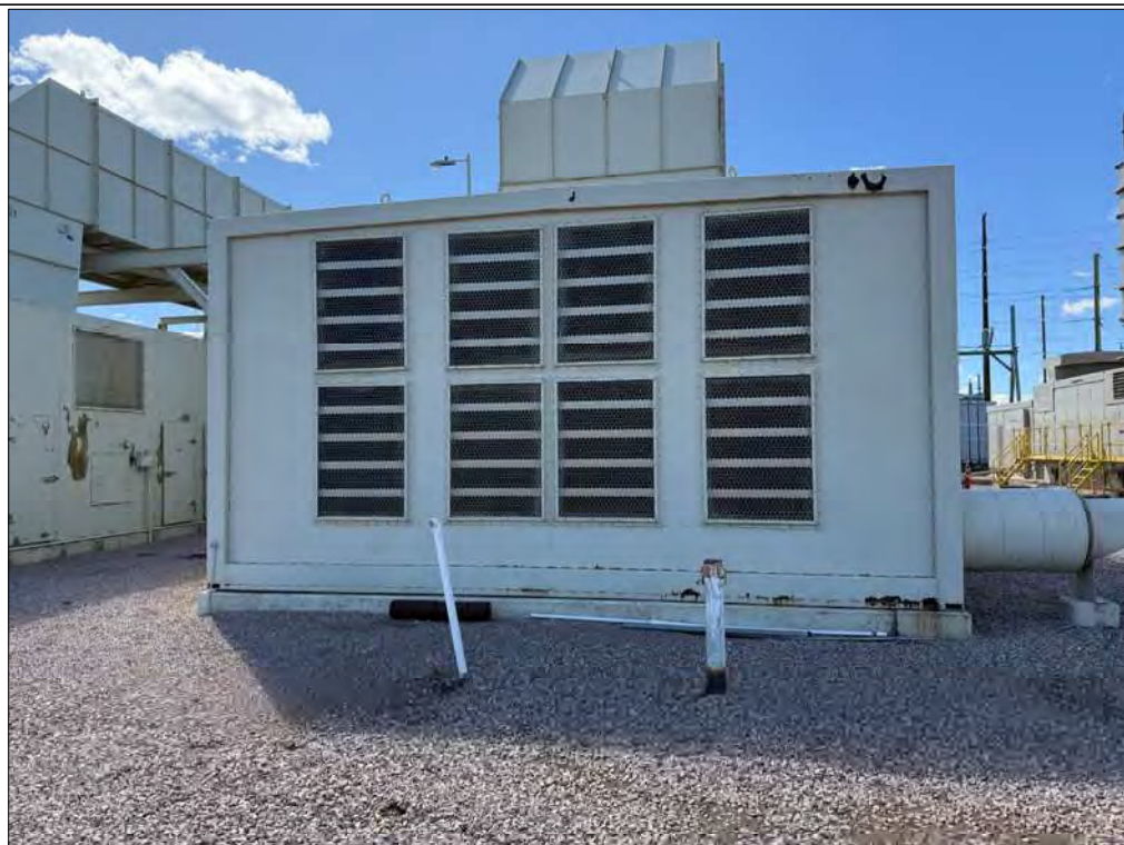
Photo 10: Piping marking potential location of UST on the east end of each of the natural gas-fired generators.
