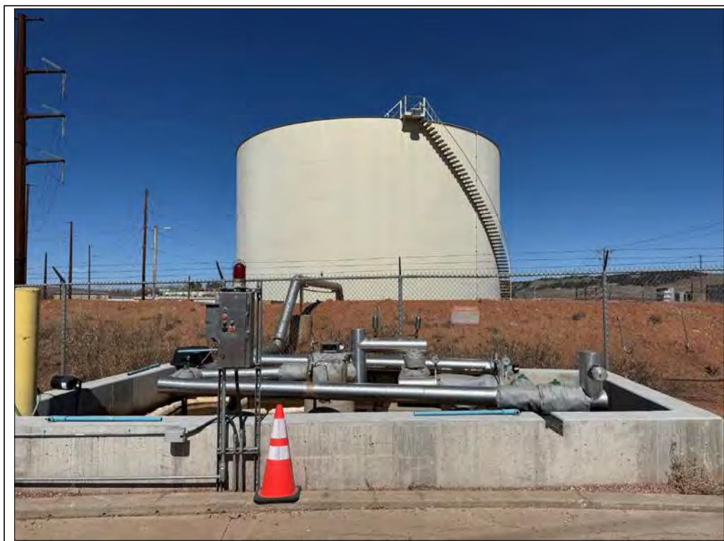
Photo 2: Fueling pad associated with 1,000,000-gallon diesel ASTs looking north.
