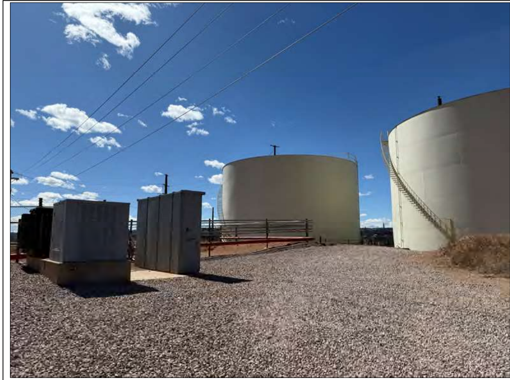
Photo 3: Pad to the east of the 1,000,000-gallon diesel ASTs looking southwest.
