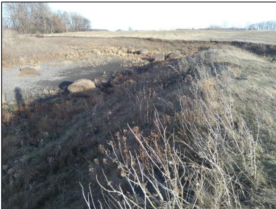
Photograph C-46: View of FFA-45S, facing east.
