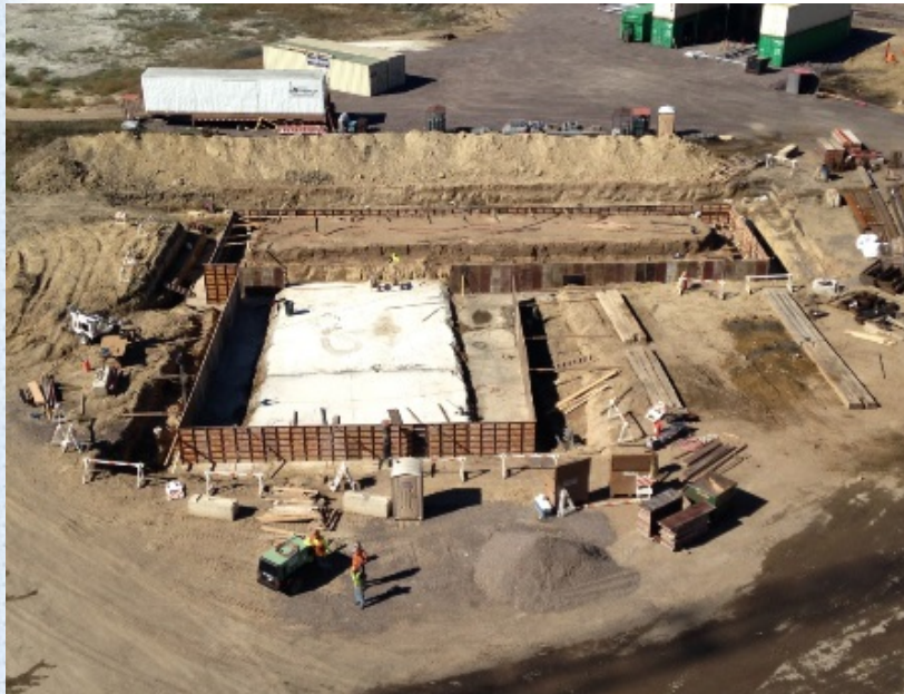
2013-10-01 Ammonia foundation formwork
