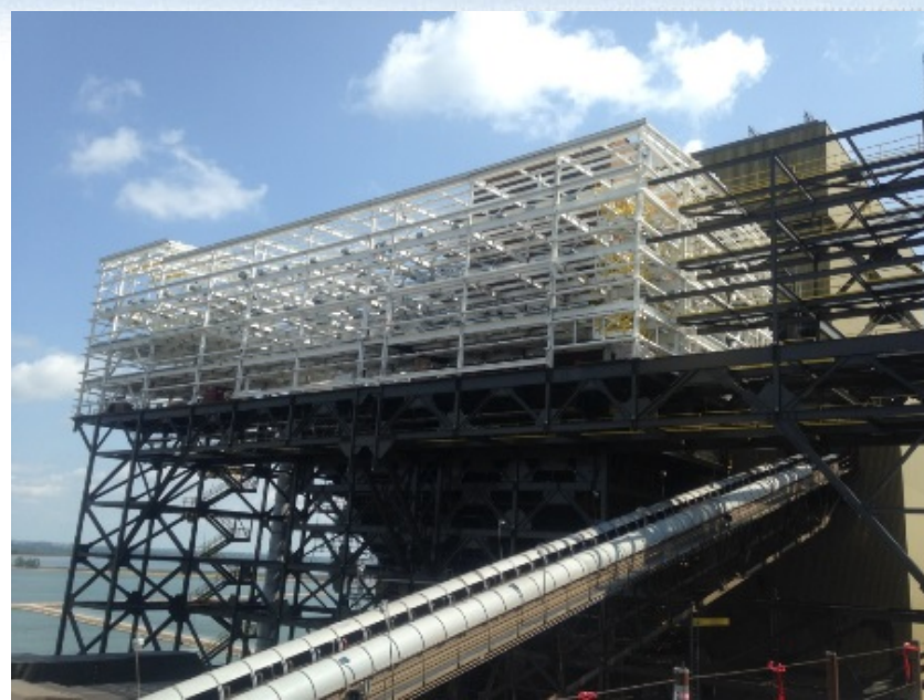
2014-08-20 Center SCR grating install
