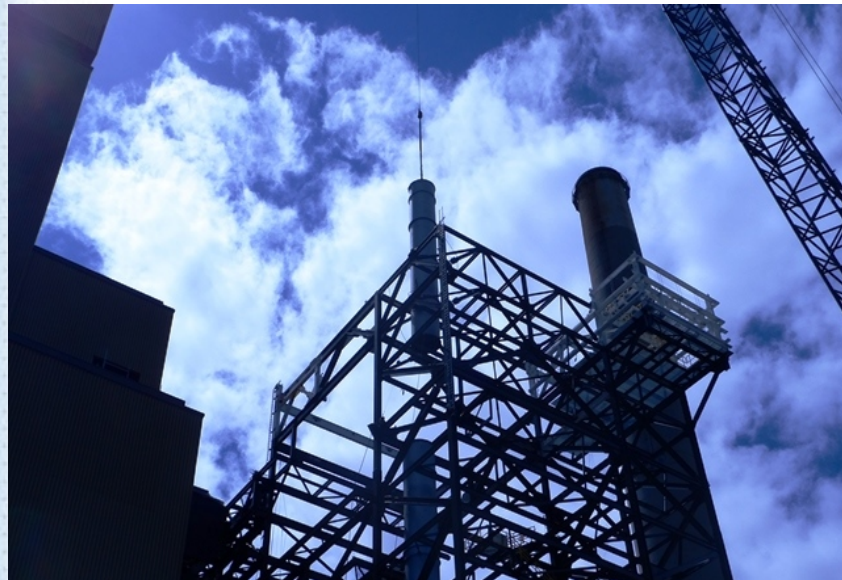
2014-05-14 Setting aux boiler stack
