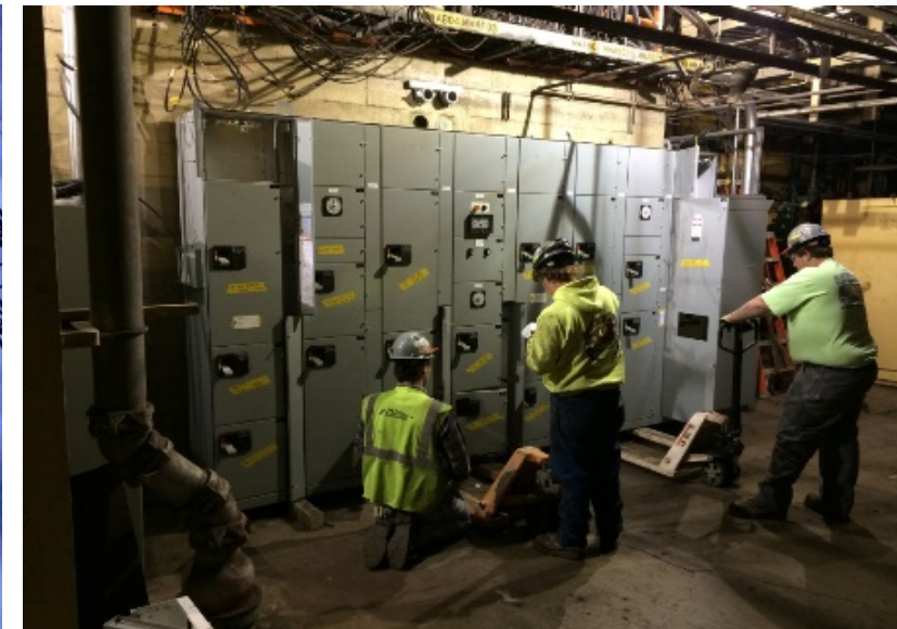
2014-05-18 Installing new DC MCC
