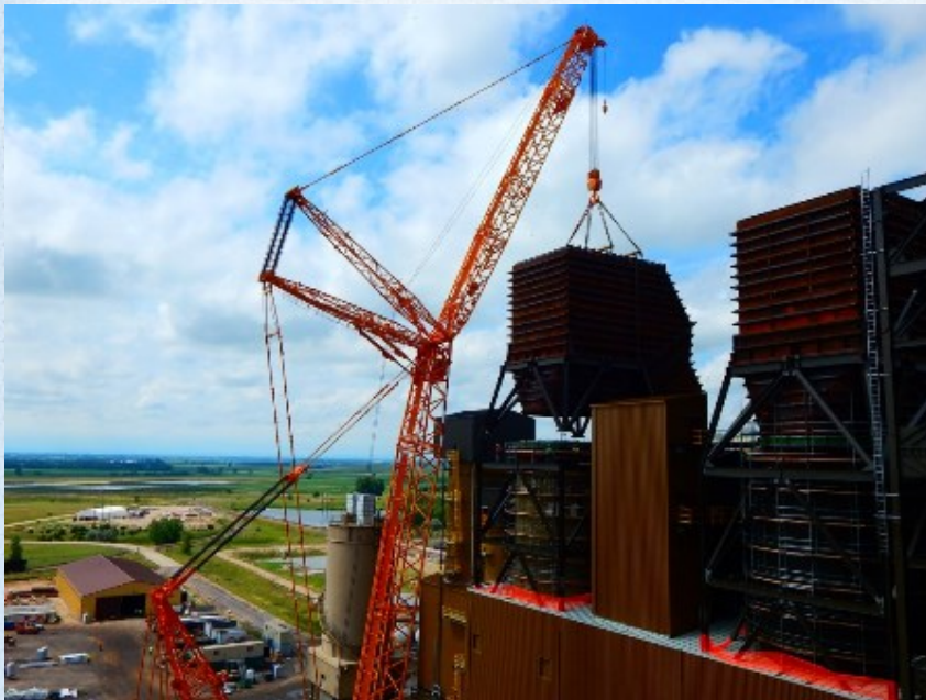
2014-08-15 Scrubber outlet transition elbow T2, heaviest lift
