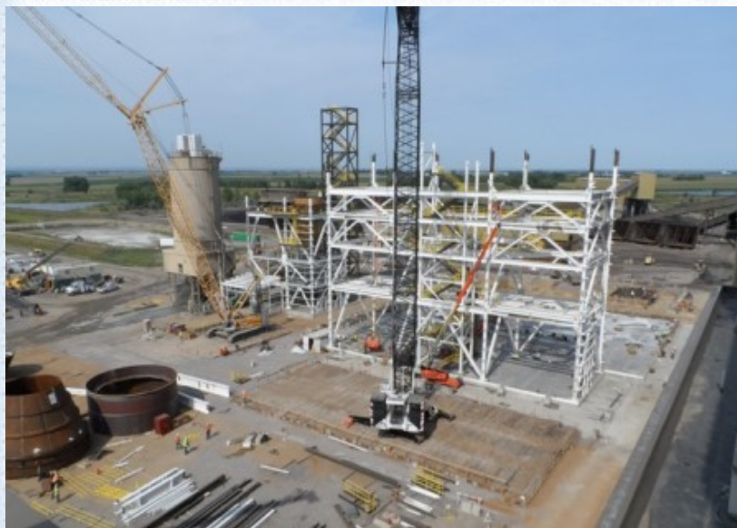
2013-08-21 Steel erection CFB, WA/PL
