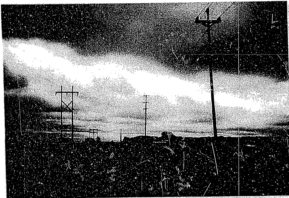
Exhibit 21.7: Westward view from Range Road showing its intersection with Highway 1804 and Perch Place. East River Cooperative's 69kV line is on the left, Oahe Electric Co-op's 13.8kV distribution line is on the right, and a farm complex is on the far right.
