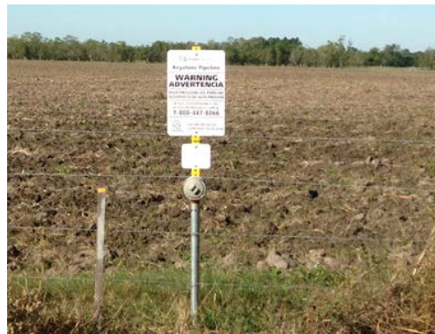
Figure 24: Typical Test Station
