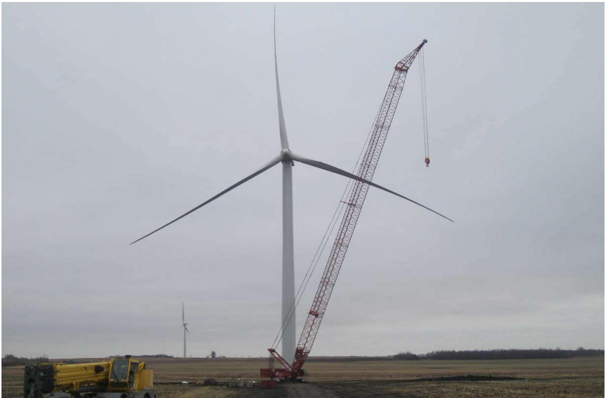
Photo: Wind tower construction west of Waverly.
