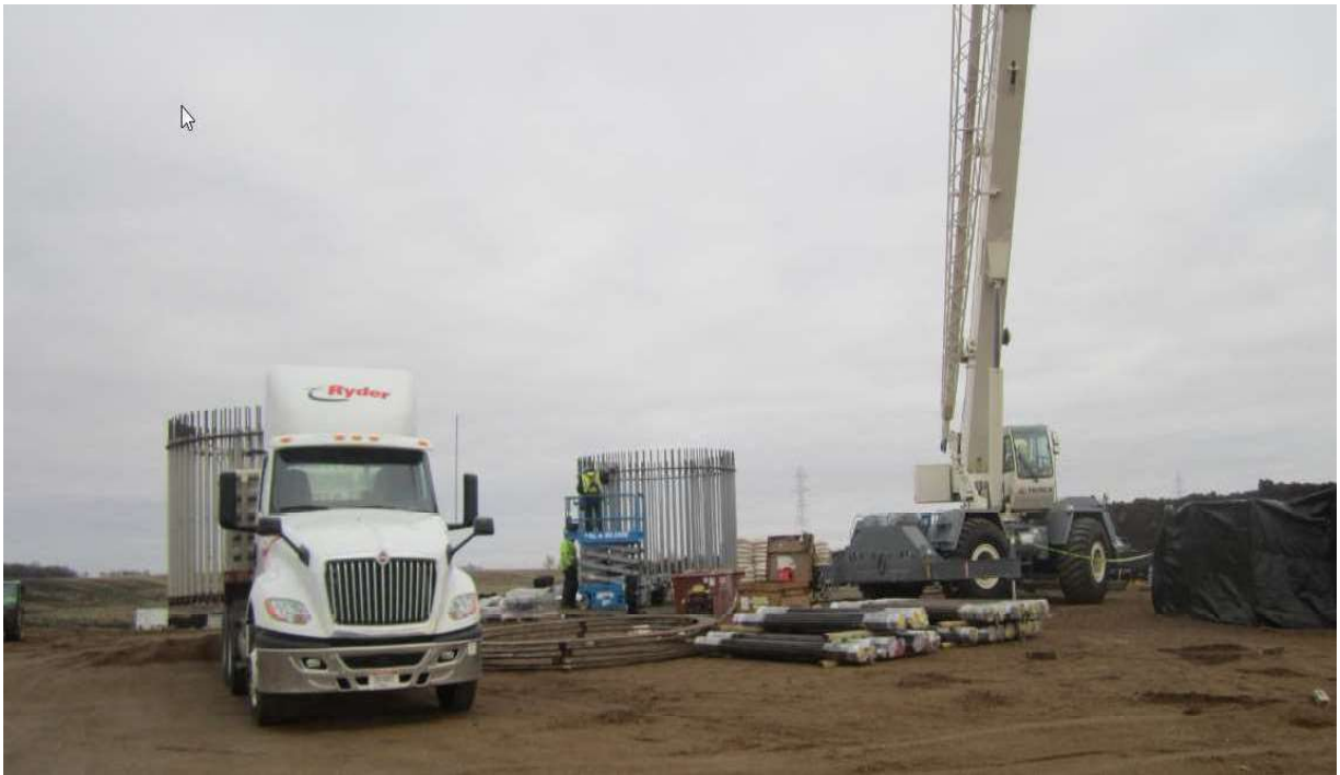
Wind tower construction by Waverly November 2019
