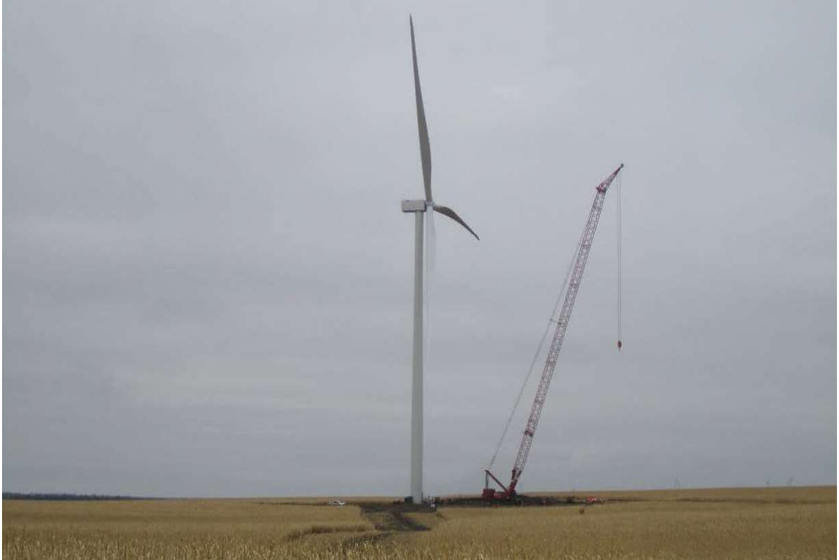
Photo: Wind tower construction west of Waverly
