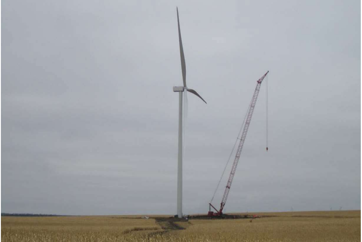
Photo: Wind tower construction west of Waverly
