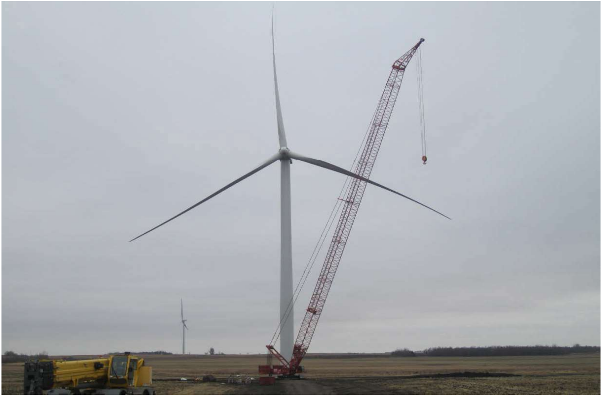
Photo: Wind tower construction west of Waverly.
