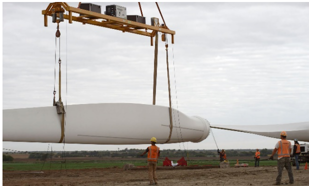
Financing and Construction
