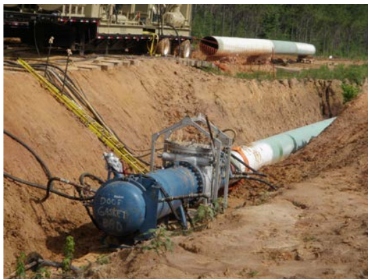
Figure 29: Drying process after hydrotest
